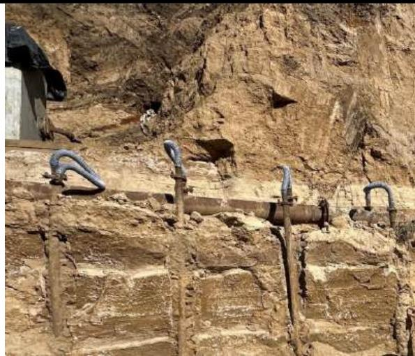
Figure 4. Drainage of the construction pit with needle filters:
